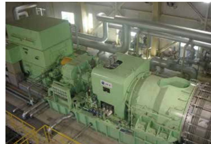
25,000kW Condensing Turbine for Biomass Power Plant, Tochigi Plant of Sumitomo-Osaka Cement Corporation
