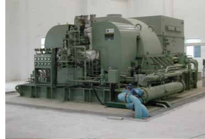
18,500kW Double Mixed steam Condensing Turbine for Cement Kiln Waste Heat Recovery Power Plant, Rui Chang Plant of Jiangxi Ya Dong Cement Corporation
