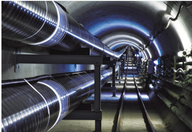
Underwater pipelines supply natural gas across the Port of Nagoya (Aichi Prefecture) to two thermal power plants.
