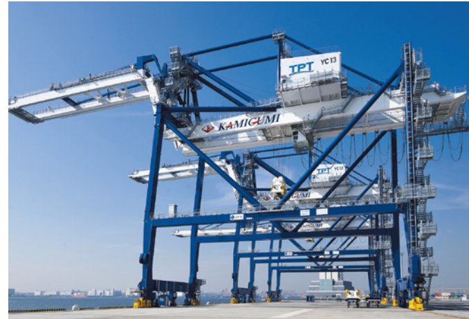
Our container cranes strengthen cargo handling operations at ports nationwide.
