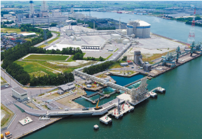
Toyama Shinko LNG Terminal (Toyama Prefecture), supporting the Hokuriku region's energy industry.
