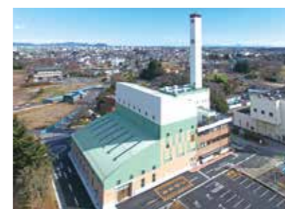
1 Tatebayashi Clean Center (incineration plant)
