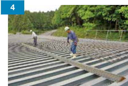
Installing reinforcing bars
