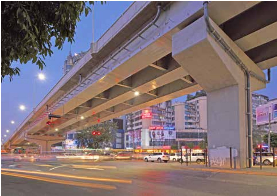
2 MyayNiGone Flyover (in Yangon) Employer: Yangon Regional Government Bridge Length: 490m Bridge Span: Span length 30 ~ 60m total 11 spans Width: 14.6m Bridge Type: 3-span Continuous box girder, etc. Steel Tonnage: 1,900 tons Completion: 2015
