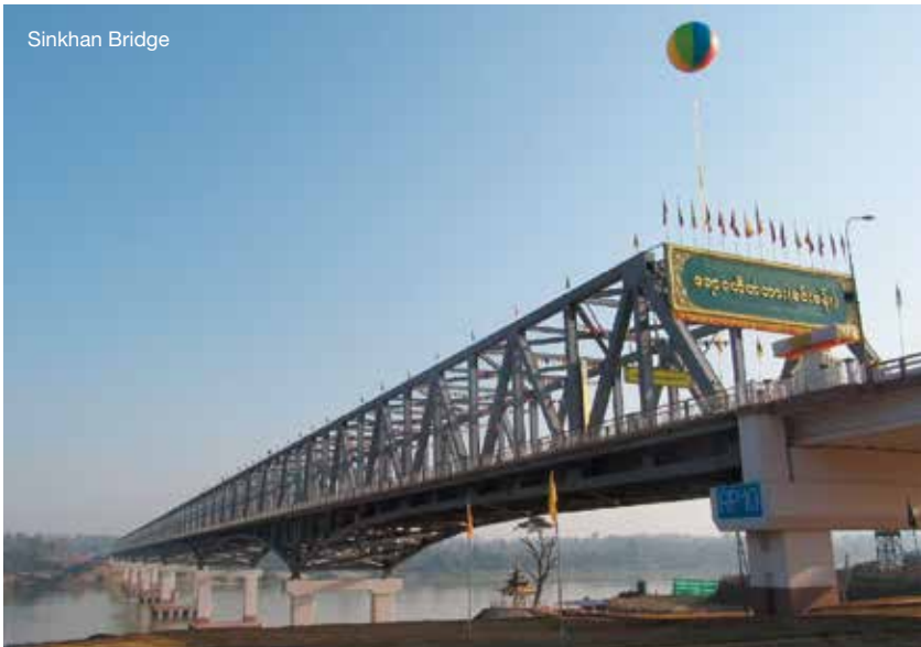
4 Sinkhan Bridge (in Kachin) 5 Marun Bridge (in Magwe) Employer: Ministry of Construction Bridge Length: 982m Bridge Span: 96.0+2@112.0m, 3@112.0m, 2@112.0+96.0m Width: (Road way) 9.1m, (Rail way) 4.3m Bridge Type: 3-span Continuous truss bridge Steel Tonnage: 9,170 tons Completion: 2012 (Shinkhan Bridge), 2013 (Marun Bridge) Feature: Combined bridge for railway/road
