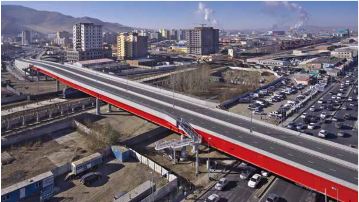
Taiyo Bridge (in Mongol) Employer : Ministry of Road and Transport Mongolia Bridge Length : 262.0m Bridge Span : 29.5+47.0+50.0+55.0+50.0+29.5m Width : 21.5m Bridge Type : 6-span continuous composite steel girder Bridge Steel Tonnage : 2,000 tons Completion : 2012 Feature : Largest Steel Bridge in Mongol, Composite Slab (River Deck) used
