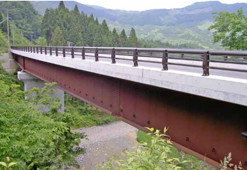
Jyougakura Bridge (in Aomori, Japan) Employer: Aomori Prefecture Bridge Length: 360m Bridge Span: 31.0+3.0+255.0+3.0+33.0+33.0m Width: 12.3m Bridge Type: 2 hinged arch bridge Steel Tonnage: 3,300 tons Completion: 1994
