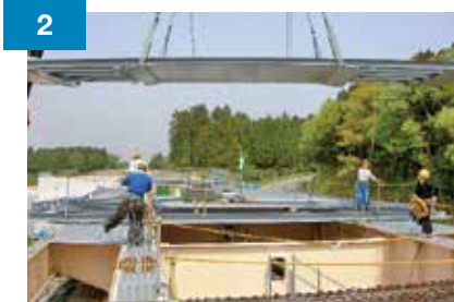
Installing and adjusting a panel
