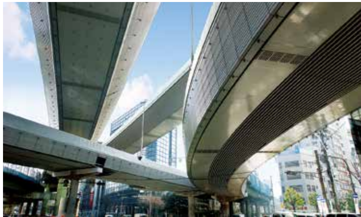
Minatomachi South Exit (in Osaka, Japan)
