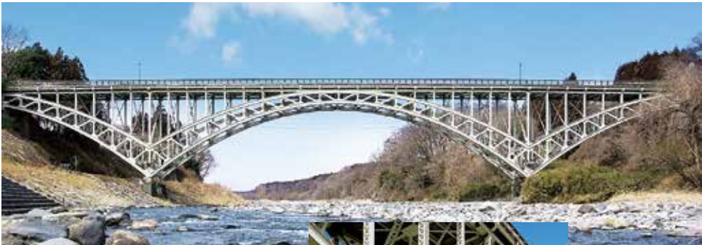
Bansui Bridge (in Tochigi, Japan)
