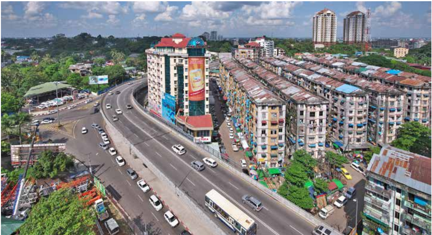
3 ShweGoneDaing Flyover (in Yangon) Employer: Yangon Regional Government Bridge Length: 481m Bridge Span: Span length 30 ~ 46m / total 12 spans Width: 14.84m Bridge Type: 4-span Continuous box girder, etc. Steel Tonnage: 1,500 tons Completion: 2013
