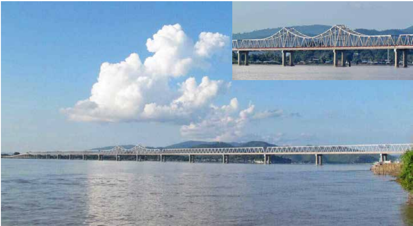
1 Htee Gyaint Bridge (in Sagaing) Employer: Ministry of Construction Bridge Length: 1,800m Bridge Span: 3@120m x 5 bridges Width: 9.42m Bridge Type: 3-span Continuous truss bridge Steel Tonnage: 9,000 tons Completion: 2015
