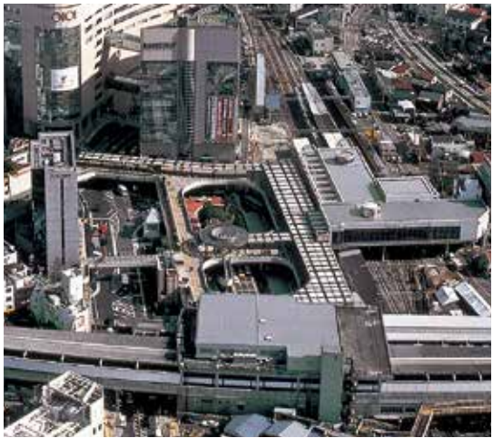
Kirari-Deck (Mizonokuchi Station Pedestrian Deck) (in Kanagawa, Japan)
