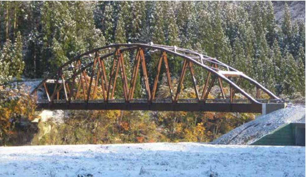
Nishibu Bridge (in Fukushima, Japan) Employer: Hokuriku Regional Development Bureau, Ministry of Land, Infrastructure, Transport and Tourism (MLIT) Bridge Length: 104m Bridge Span : 102.6m Width: 6.2m Bridge Type: Langer truss Steel Tonnage: 345 tons Completion: 2013
