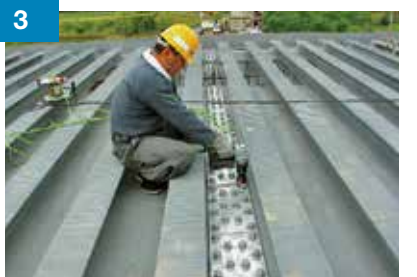
Joining a bottom plates at a site (one-side bolting)
