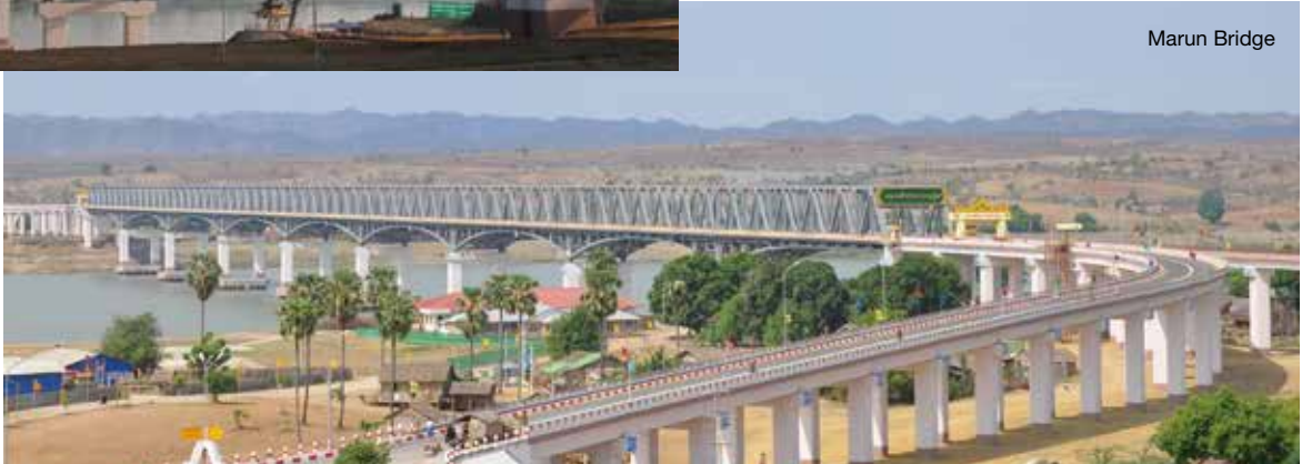
4 Sinkhan Bridge (in Kachin) 5 Marun Bridge (in Magwe) Employer: Ministry of Construction Bridge Length: 982m Bridge Span: 96.0+2@112.0m, 3@112.0m, 2@112.0+96.0m Width: (Road way) 9.1m, (Rail way) 4.3m Bridge Type: 3-span Continuous truss bridge Steel Tonnage: 9,170 tons Completion: 2012 (Shinkhan Bridge), 2013 (Marun Bridge) Feature: Combined bridge for railway/road
