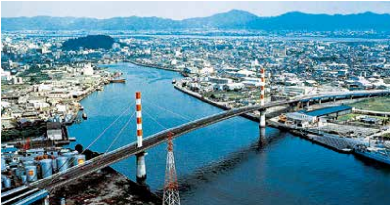
Suehiro Bridge (in Tokushima, Japan)
