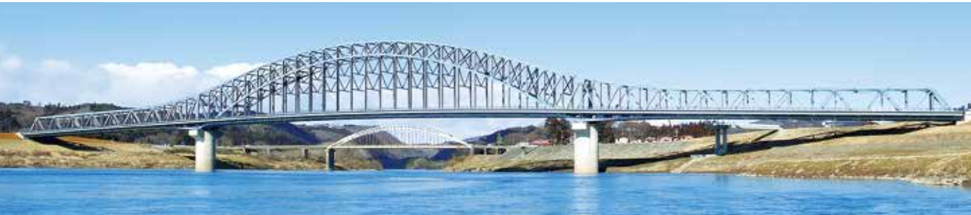
Shinkitakami Bridge (front) (in Iwate, Japan)
