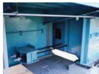
Bridge collapse preventing system, shoe replacement
