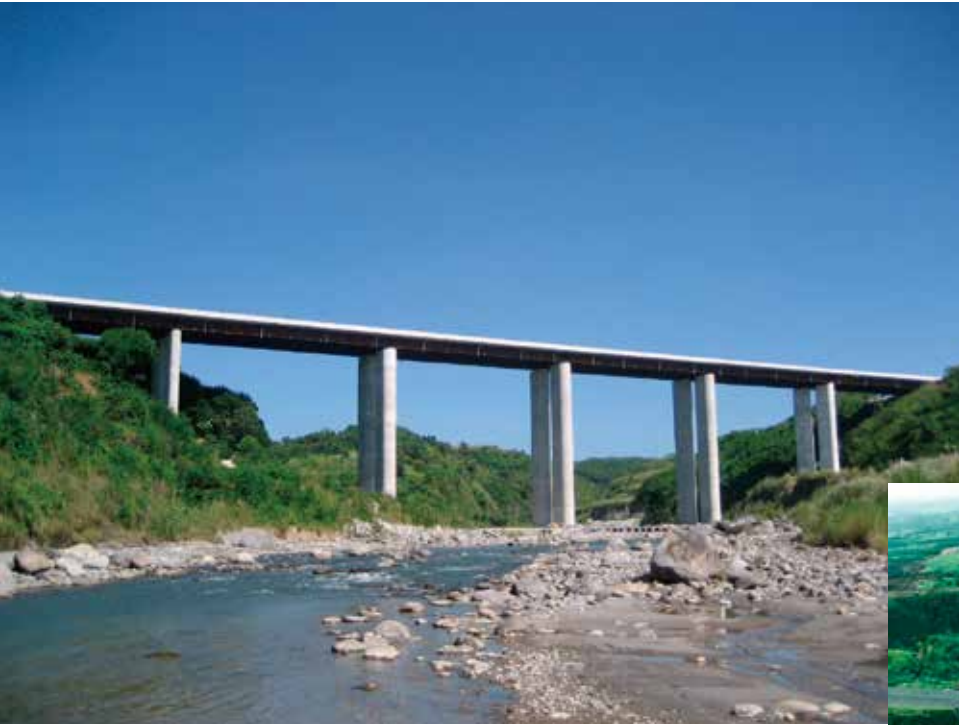
Gumain Bridge (in Philippines) Employer : Bases Conversion and Development Authority Bridge Length : 360.0m Bridge Span : 5.3+4@60.6+59.3m Width : 23.0m Bridge Type : 6-span continuous small-number main girder Bridge Steel Tonnage : 1,930 tons Completion : 2008 Feature : Weather-resistant steel used
