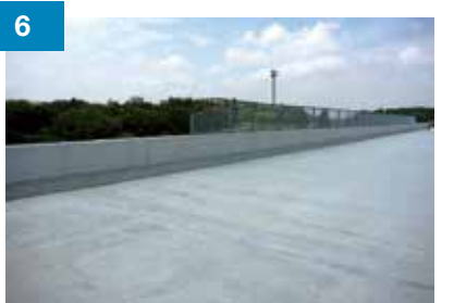
Completion of work
