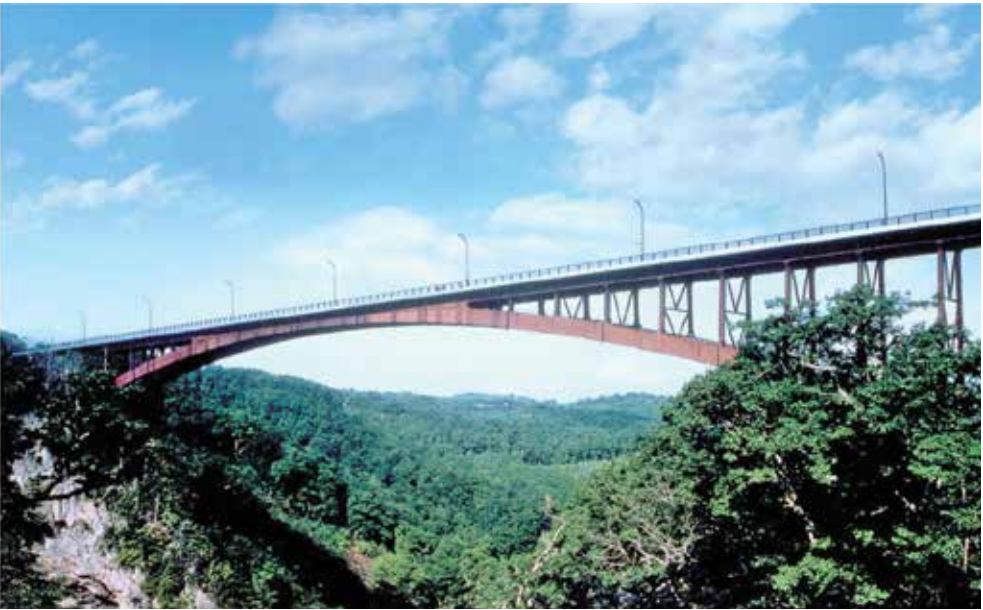
Jyougakura Bridge (in Aomori, Japan) Employer: Aomori Prefecture Bridge Length: 360m Bridge Span: 31.0+3.0+255.0+3.0+33.0+33.0m Width: 12.3m Bridge Type: 2 hinged arch bridge Steel Tonnage: 3,300 tons Completion: 1994
