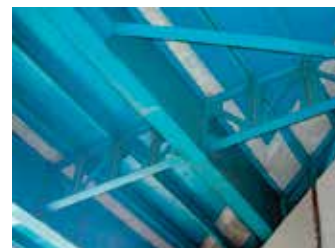
Deck reinforcement through girder addition and steel plate bonding
