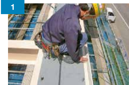
Sealing a upper flange
