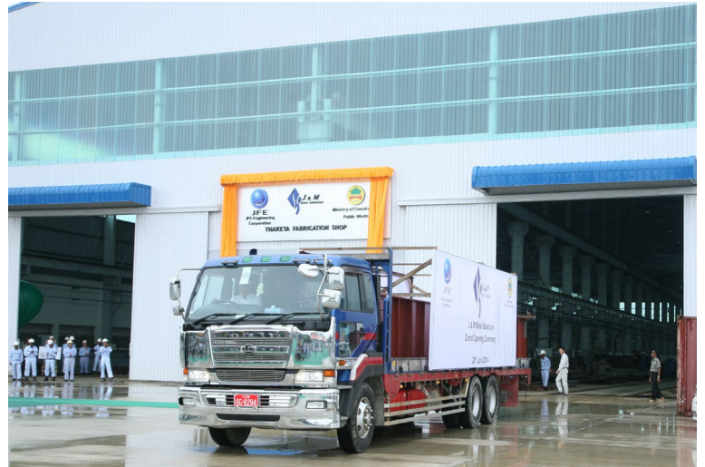
□ First shipment of a bridge block
