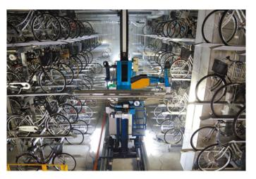
The low-footprint CycleTree® automated parking system outside Sagami-Ono Station (Kanagawa Prefecture).
